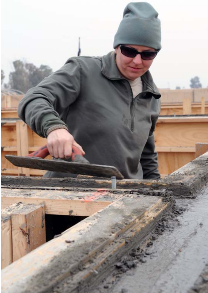
Senior Airman Carol Clements, 506th Expeditionary Civil Engineer Squadron structures technician, levels concrete while setting walls on a new building project in January. (U.S. Air Force photo/SSgt Tabitha kuykendall)
